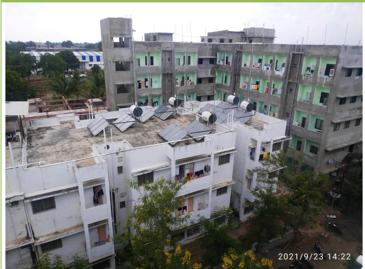
Solar Water Heating System- 21450litres/day- Hostel
